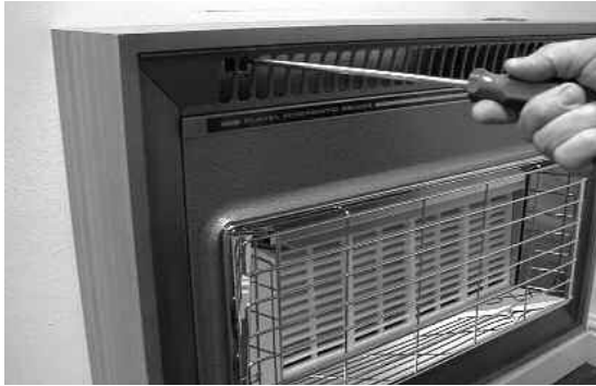
Fig. 10 Removing the Upper Outer Case Fixing Screws
