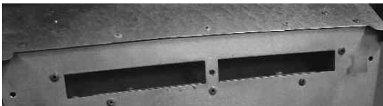
Fig 4 - Flue Restrictor Baffle Not Fitted
